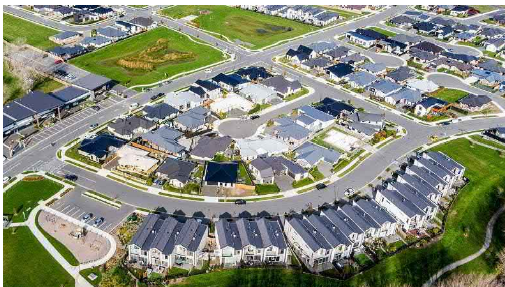
Image 4: Aerial photograph of the Silverstream subdivision, Kaiapoi
