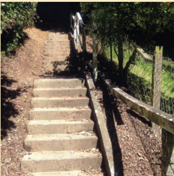
Figure 4.2 Walkway between Hazelwood Ave and South Karori Rd, broken railing, December 2013.
