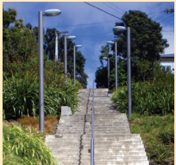
Figure 4.3 Walkway with lighting and metal rails, part of Drummond St, Mt Cook, November 2013.
