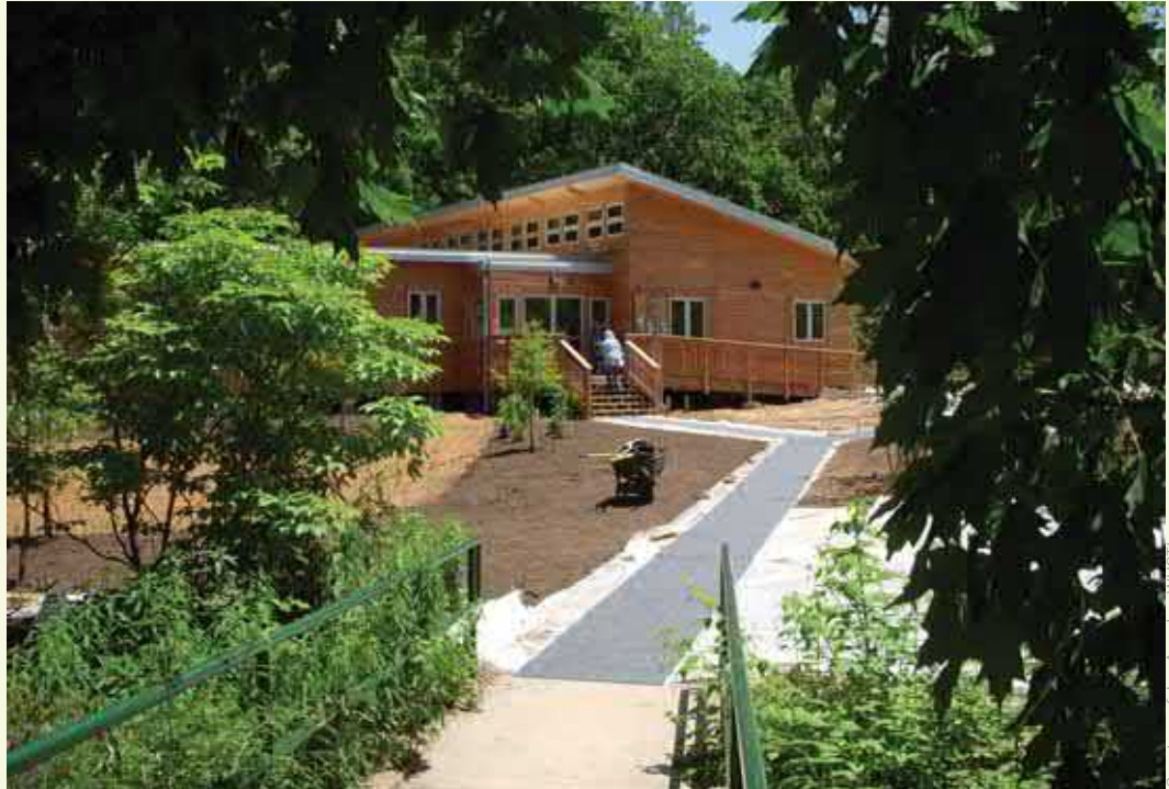
Tyson Living Learning Center irrigates its landscape with greywater collected from building sinks.
