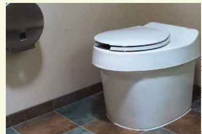
The waterless toilet by Clivus Multrum helps reduce overall water requirements.
