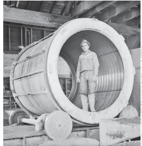
Six foot diameter sewer pipe, 1935.
